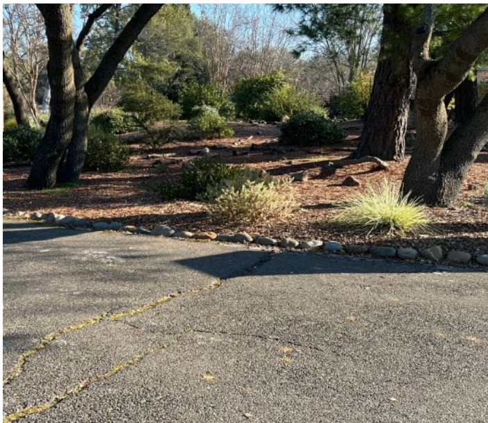
Roots of mature shade trees have cracked this asphalt driveway.
