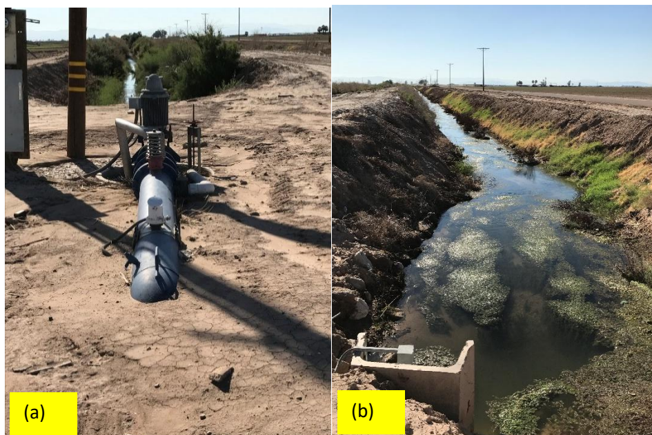
Fig. 3. Tailwater recovery system in Imperial Valley. The figure shows (a) a semi-permanent tailwater recovery system (pump and accessories) and (b) an open drainage canal as its water supplier.
