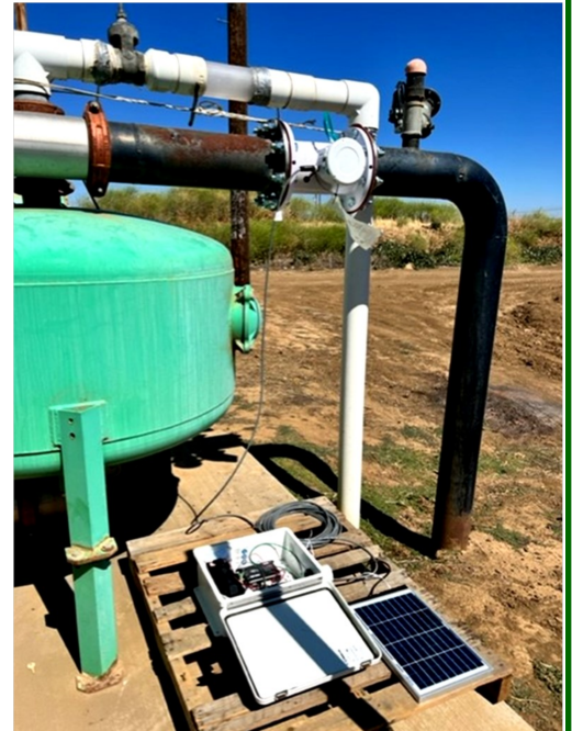
Figure 4. Finished layout of the flow meter and dataloggers that were established at the main pump from the 2022 study.
