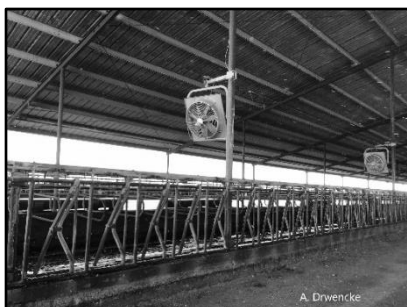
Fig. 2: Fans placed so that they cool cows at the bunk; moving air over wet animals removes more heat than when they are dry and means we need less soaking overall.
