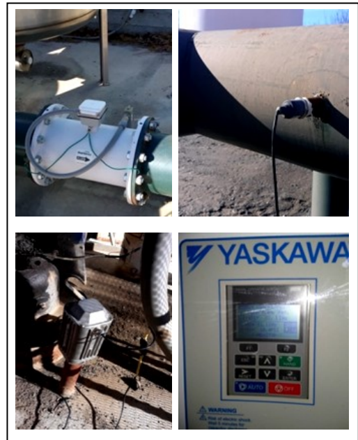
Figure 3. Magnetic flow meter (upper left), pressure transducer (upper right), acoustic groundwater level sensor (lower left), and VFD digital control panel (lower right).
