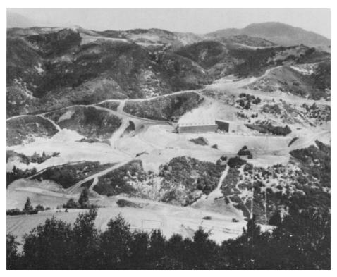
Geothermal power plants (above and opposite) with the associated site disturbances by drillpads, steam transmission lines, roads, and electric power at The Geysers, northern California. (Photos by Craig Martz.)
