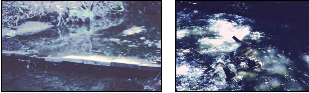
**Figure 37:** The first Stream Channel Improvement practice used a “Hewlett Ramp” design to confine high flows that scour deeper pools to improve habitat for steelhead and coho salmon. Designed by Prunuske Chatham, Inc and Trout Unlimited.
