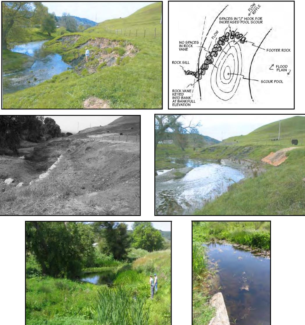
**Figure 38:** A recent Stream Channel Improvement practice in Walker Creek watershed implemented using J-hook instream enhancement techniques before the project in 2003 (top left), practice design (top right), during and following installation (second row), and five years later with the intended deep pools for aquatic species and well vegetated, stable streambanks (bottom). Designed by Prunuske Chatham, Inc. Photos by STRAW.
