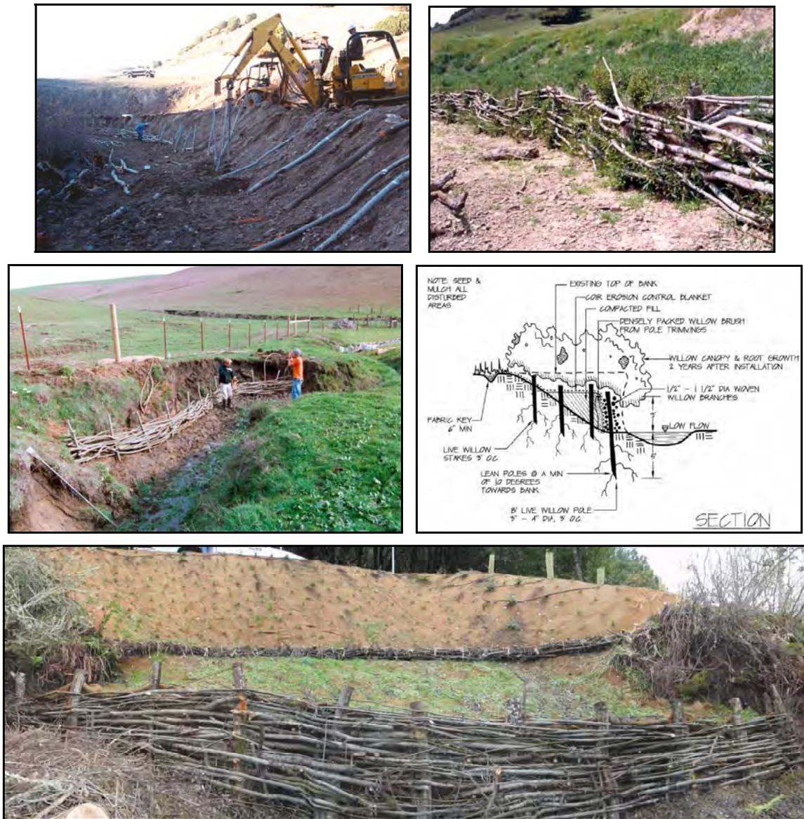
**Figure 36:** An example of the first willow walls constructed in 1990 in the Walker Creek Watershed (top), another later example constructed in 1994 (middle left), a recent design specification (middle right), and a recently constructed willow wall stabilizing the streambank toe below a threatened ranch road with willow fascine and revegetation using native grass seed, sedge/rush plugs, and shrubs in 2008 (bottom). Designs by Prunuske Chatham, Inc.
