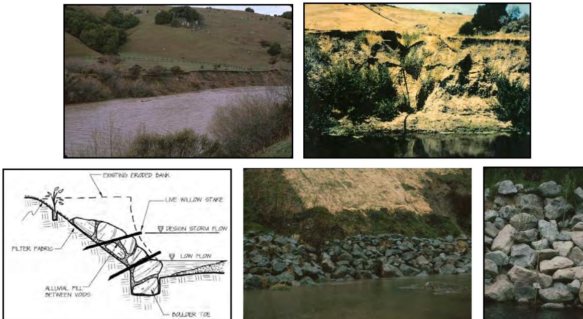
**Figure 35:** One of the first vegetated boulder revetment techniques adapted for the Streambank Stabilization practice at “one of the worst actively eroding streambanks” in Marin County before the project in 1985 (top), practice design and following installation with willow sprouts barely visible (bottom). Designed by Prunuske Chatham, Inc.
