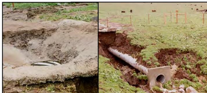
Sediment plugged inlet caused failure of Water Control Structure.
