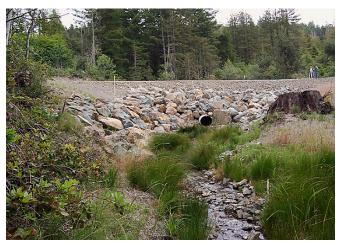
**Figure 19.** This reconstructed stream crossing on an all-season road used for hauling timber illustrates many desired design features. The culvert is sized to accommodate 100-year storm flows plus debris and sediment. It is located at the base of the road fill at the elevation of the channel to prevent scour. The face of the crossing fill is armored with rock. The road has a critical dip to prevent diversion and is surfaced with gravel. *Photo:* Richard Harris.
