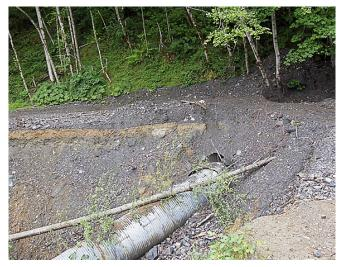
**Figure 1.** Culverted stream crossings may plug during storms. Diverted stream flow then crosses the road and erodes the fill slope. *Photo:* Richard Harris.
