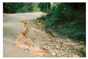
**Figure 9.** This ditch and road surface erosion was caused by inadequate spacing of ditch relief culverts. *Photo:* Susie Kocher.
