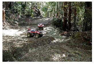
**Figure 12.** Water bars and straw mulch have been installed on this seasonal road prior to the onset of the rainy season. Water bars drain road surface runoff to prevent erosion. They will be removed when the road is put back in use. *Photo:* © Angela Wilson; used with permission.
