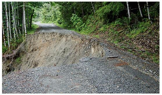
Figure 3. Stream undercutting at the base of the slope below the road caused this landslide. *Photo:* Richard Harris.
