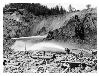
**Figure 2.** Hydraulic mining, 1860–1870, Trinity County. Streams were diverted through flumes, ditches, and pipes to monitors (nozzles) to wash gold-bearing gravels into sluce boxes for separation of the gold. *Source:* Eastman's Originals Collection Group 117, Special Collections, University of California Library, Davis, reprinted with permission.
