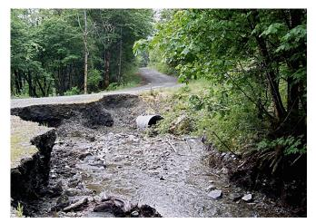
**Figure 18.** This culvert plugged with debris during a storm. Although it is still in place, the swirling water and debris caused extensive erosion of the road and the adjacent old log landing. This type of failure is common on older "legacy" roads where crossings were not adequately designed to pass 100-year flows plus debris and sediment. In many cases, the culvert will be displaced and transported downstream. *Photo:* Richard Harris.
